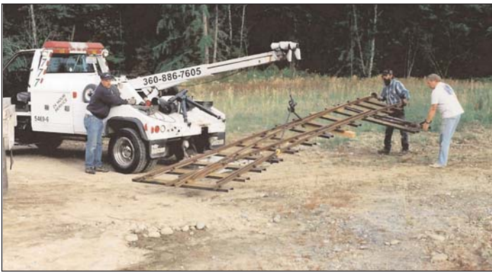
Lifting a switch off of a flat bed.
