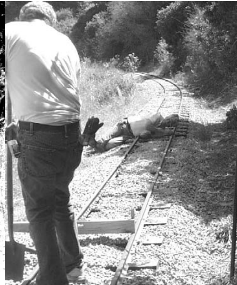
Figure 1-8: Sighting from peep sight over rabbit block to sight board
