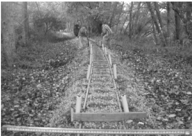
Figure 1-9; Track leveled with track jacks
