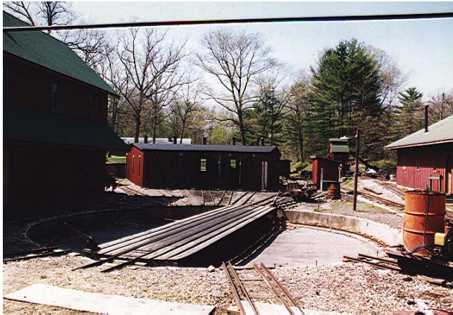
This 30' turntable serves a 5 stall roundhouse. The machine shop is at right. To the left of the turntable is where the boiler shop caught fire. In the distance between the roundhouse and the machine shop, the small green roof marks the scale coaling tower. Photo:
