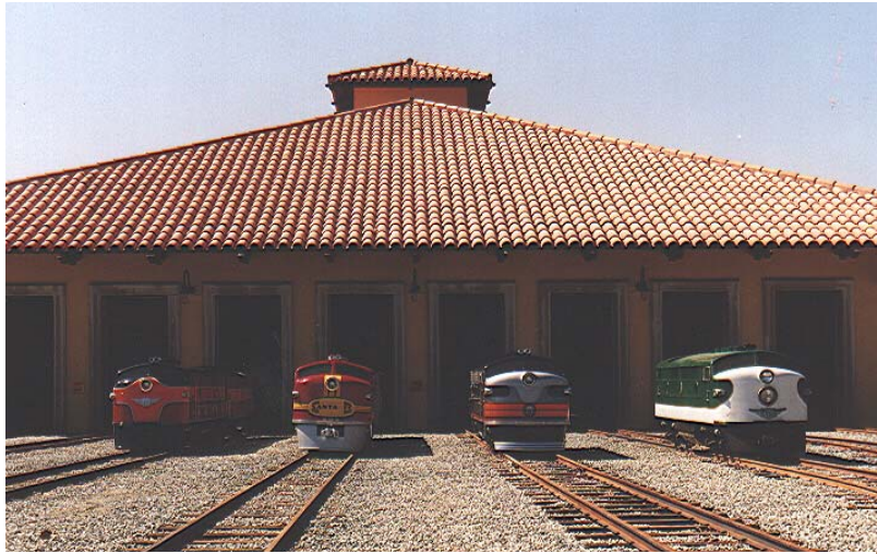
The car barn / roundhouse has a very Southwestern (US) feel to it with the Spanish tile roof. A very railroad-like atmosphere was achieved in the interior with the use of large timber trusses and beams.
